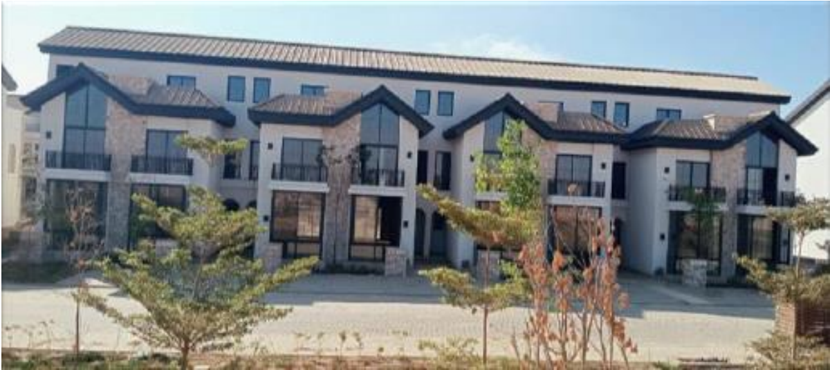
Plot 3 (elevation repainting)
