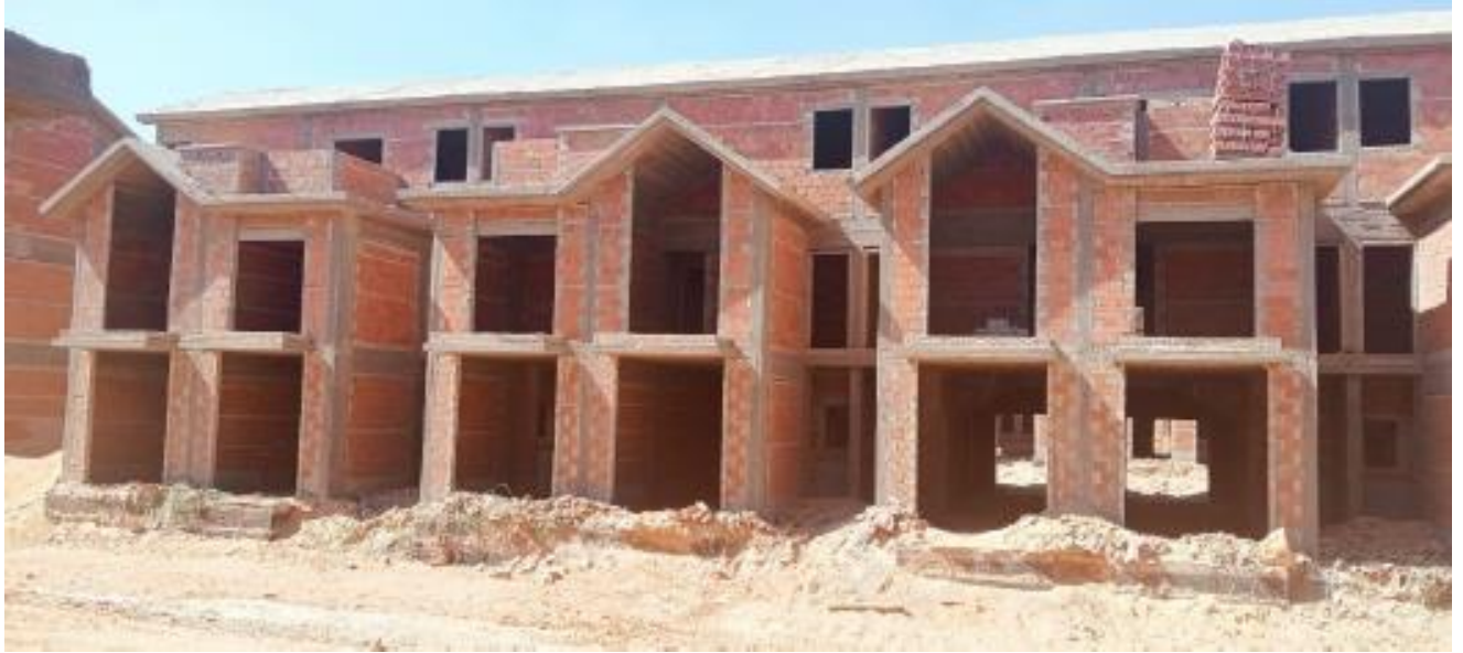
Plot 36 (external finishes – blockwork)
