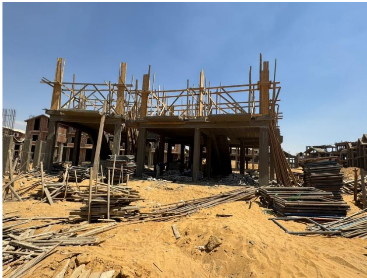
Plot 60 (1st floor columns)
