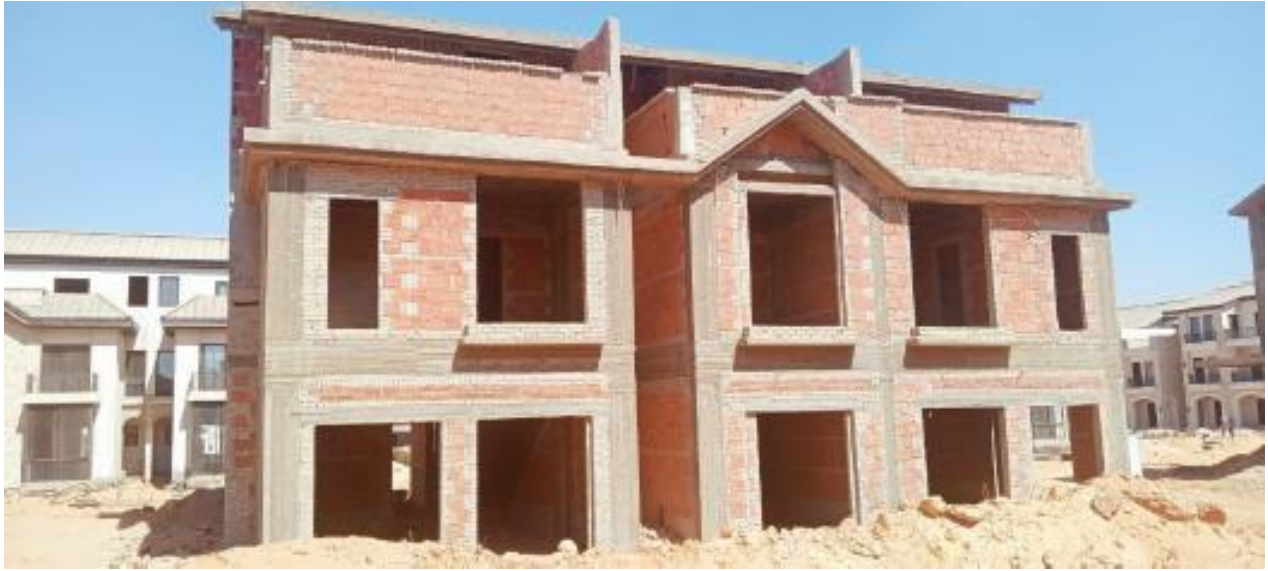
Plot 35 (external finishes – blockwork)
