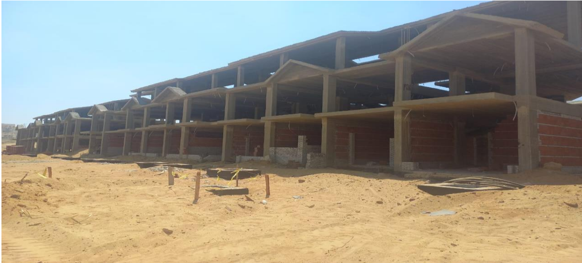
Plot 11 (external finishes – blockwork)
