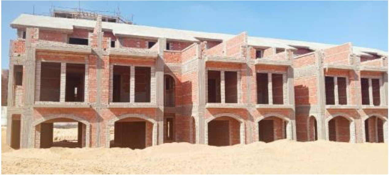
Plot 20 (external finishes – blockwork)
