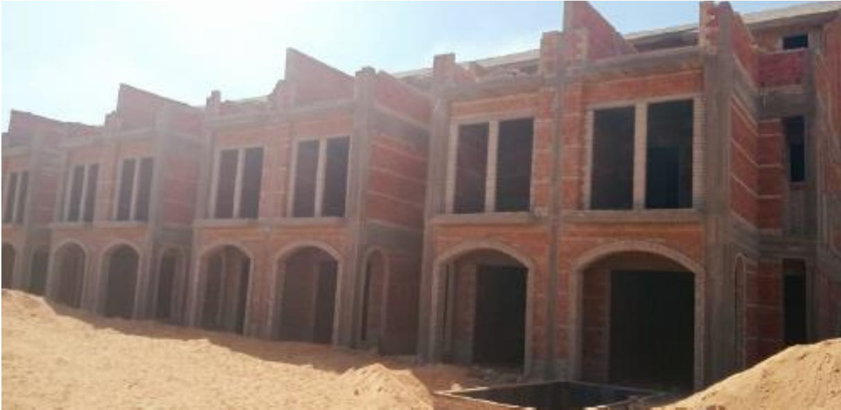
Plot 18 (external finishes – blockwork)
