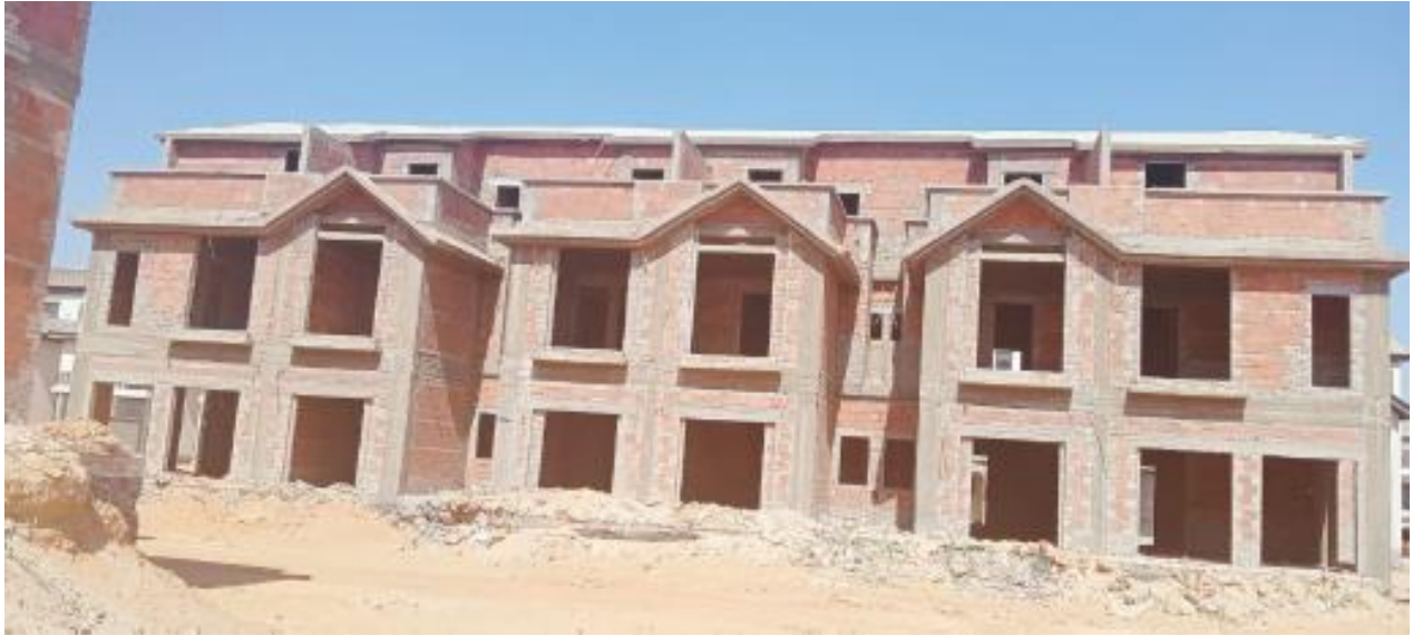
Plot 45 (external finishes – blockwork)
