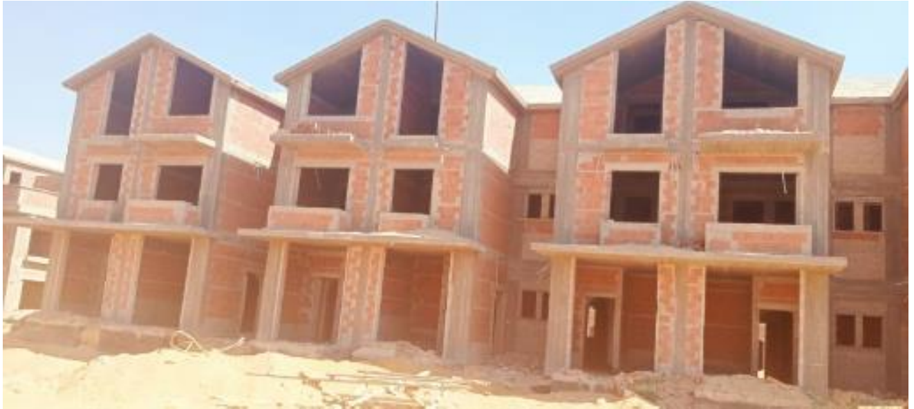
Plot 46 (external finishes – blockwork)
