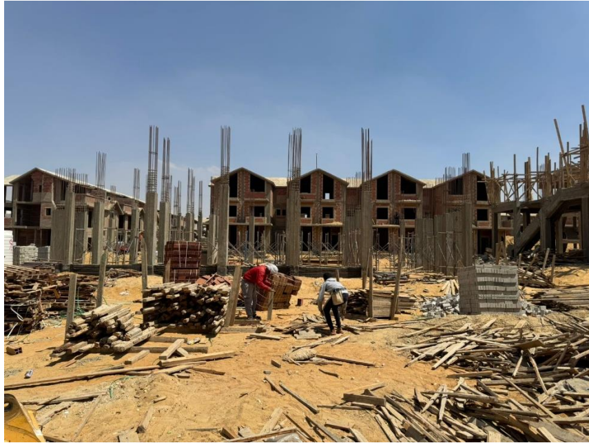
Plot 61 (first floor slab)
