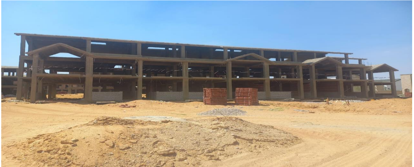
Plot 10 (external finishes – blockwork)
