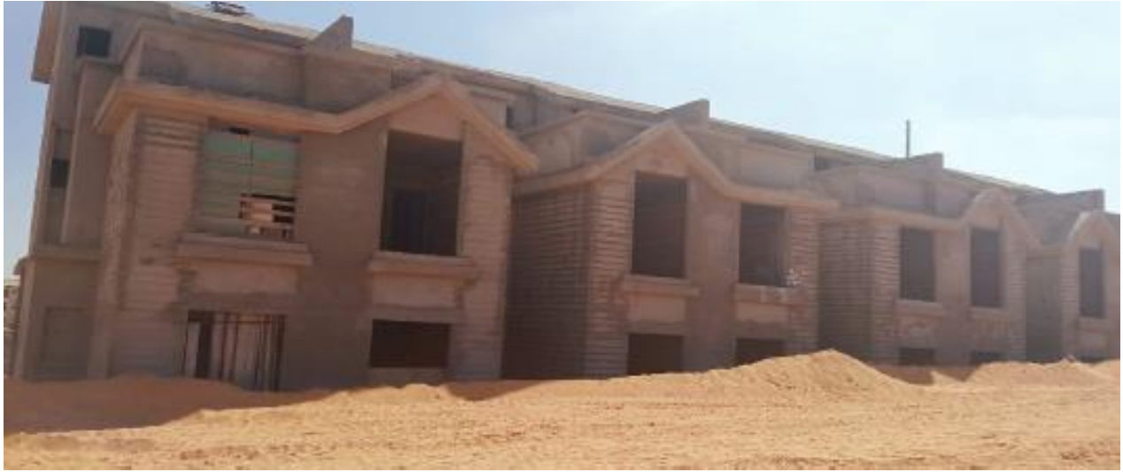
Plot 25 (external finishes – plaster)
