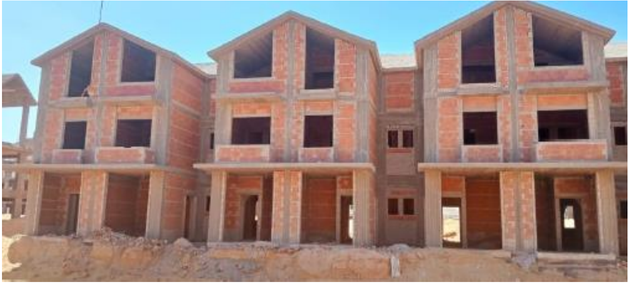
Plot 29 (external finishes – blockwork)
