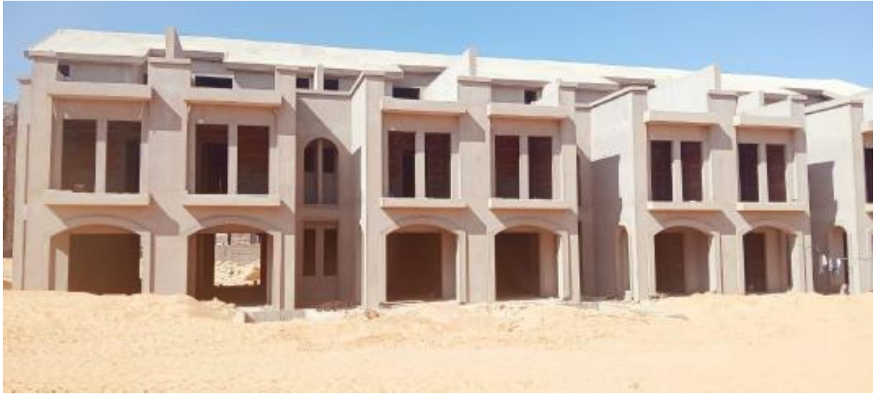
Plot 23 (external finishes – plaster)
