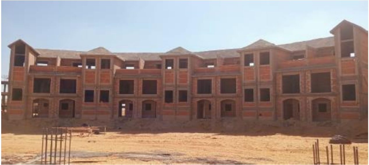
Plot 31 (external finishes – blockwork)
