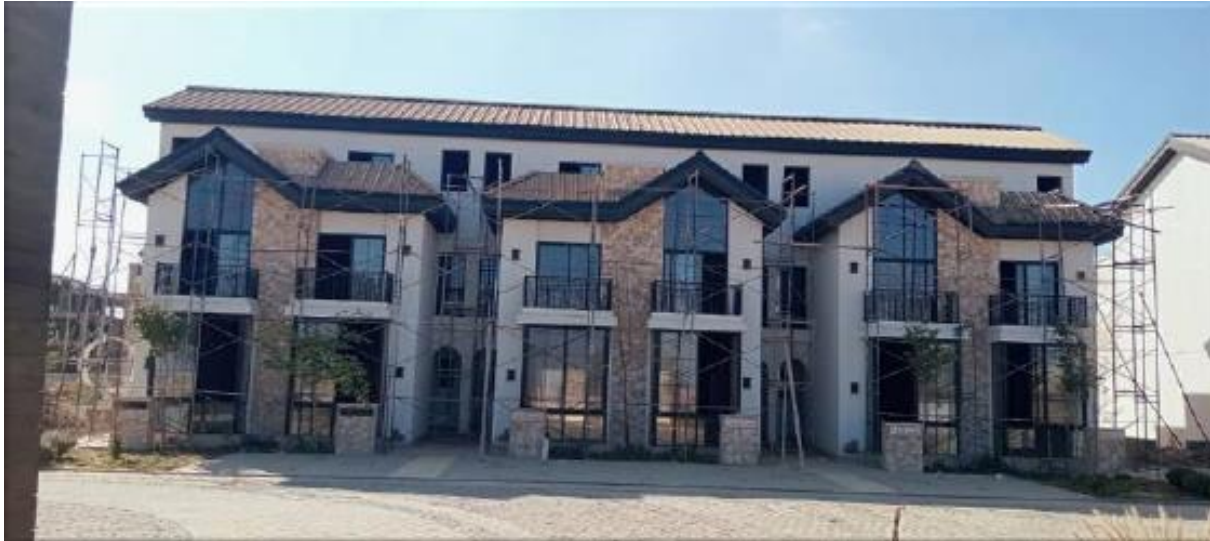
Plot 1 (elevation repainting)
