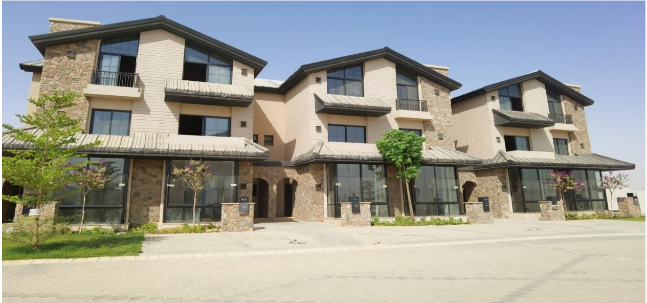
Plot 24 (elevation repainting)
