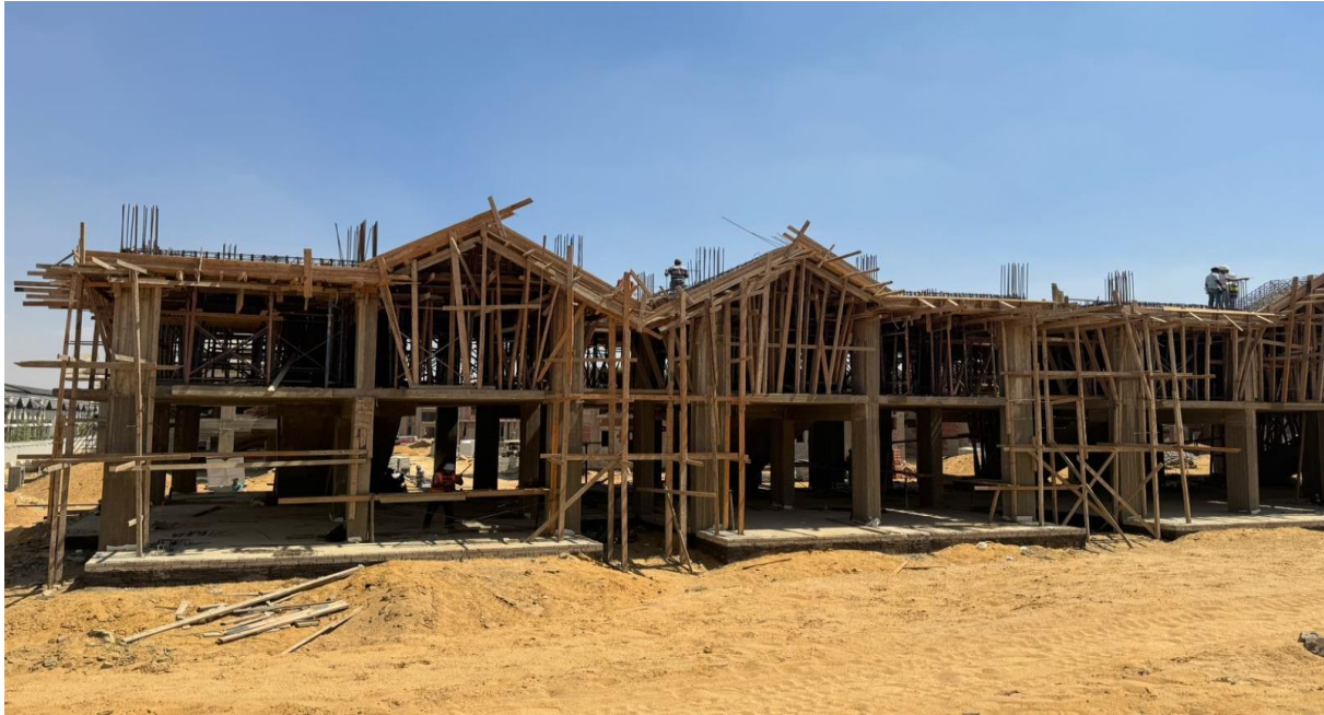
Plot 26 (first floor Slab)
