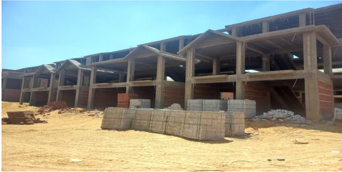
Plot 33 (external finishes – blockwork)
