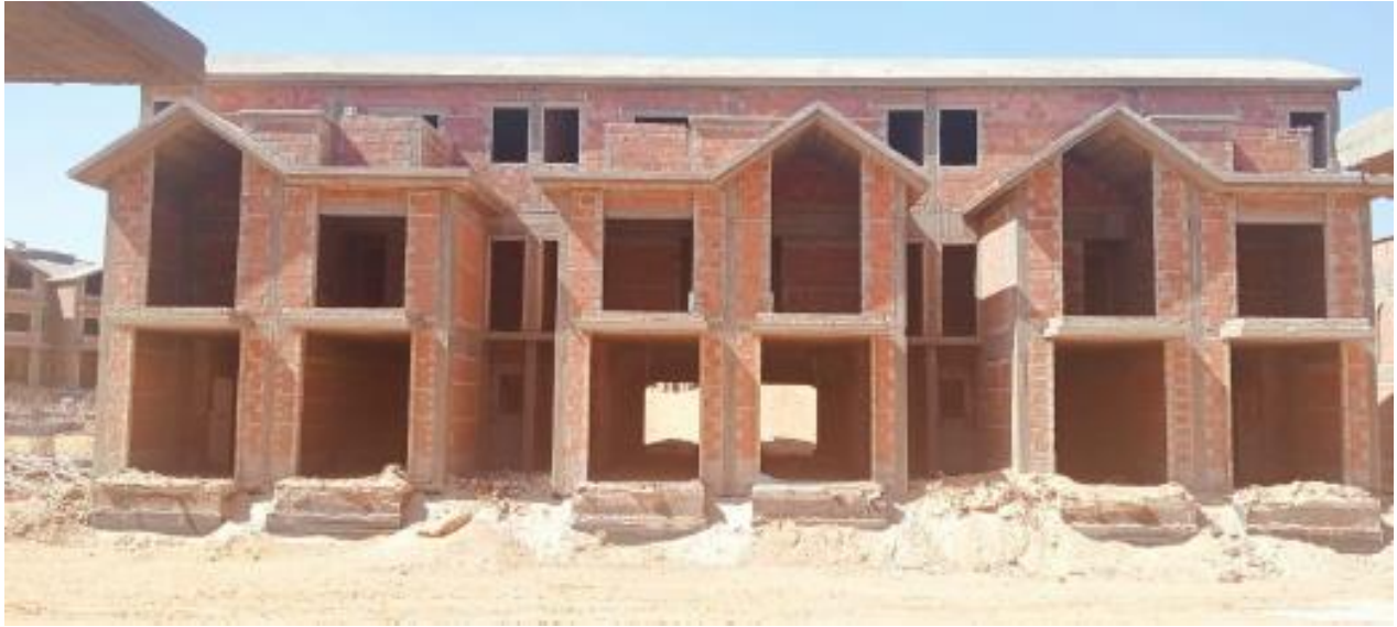
Plot 37 (external finishes – blockwork)
