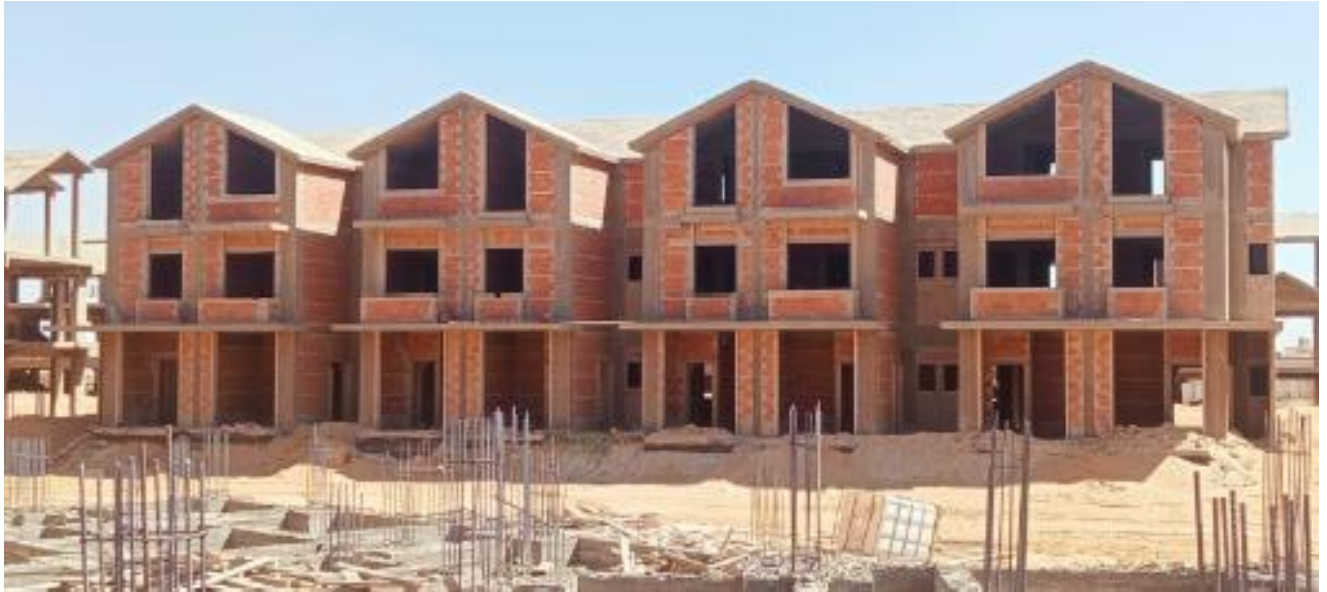
Plot 32 (external finishes – blockwork)
