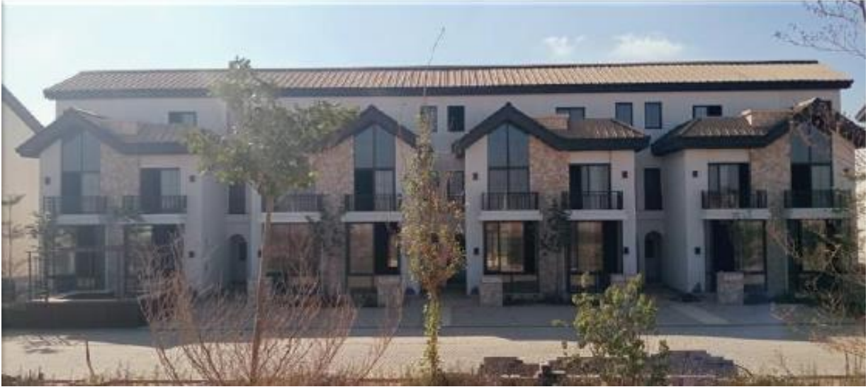
Plot 2 (elevation repainting)
